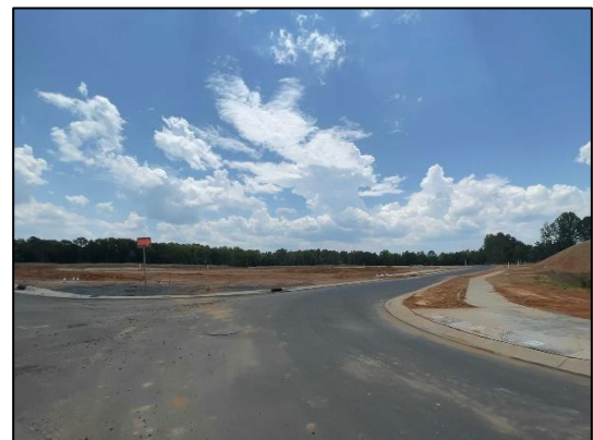
Single-family neighborhood under construction to east off Finley Road
