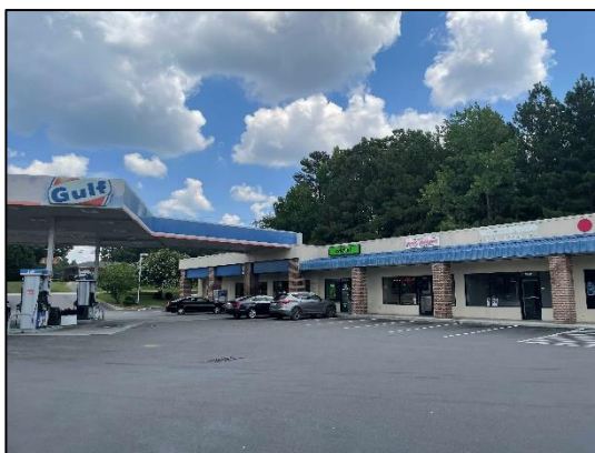
Convenience store adjacent to northwest corner of site
